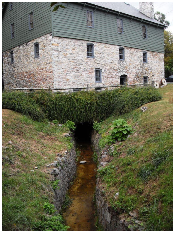
Burwell-Morgan Mill. Source: NSVRC, 2013
