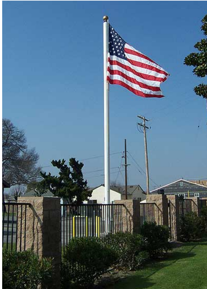
Example of a well-designed flag pole WCF
