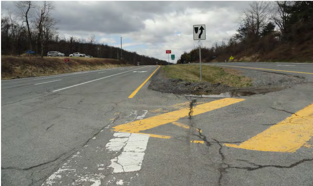
Sight Distance looking east from crossover
