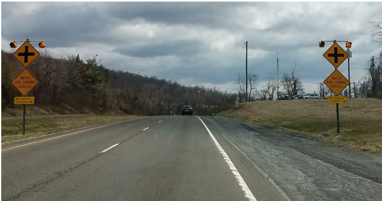
Route 7 eastbound crest vertical curve hiding intersection
