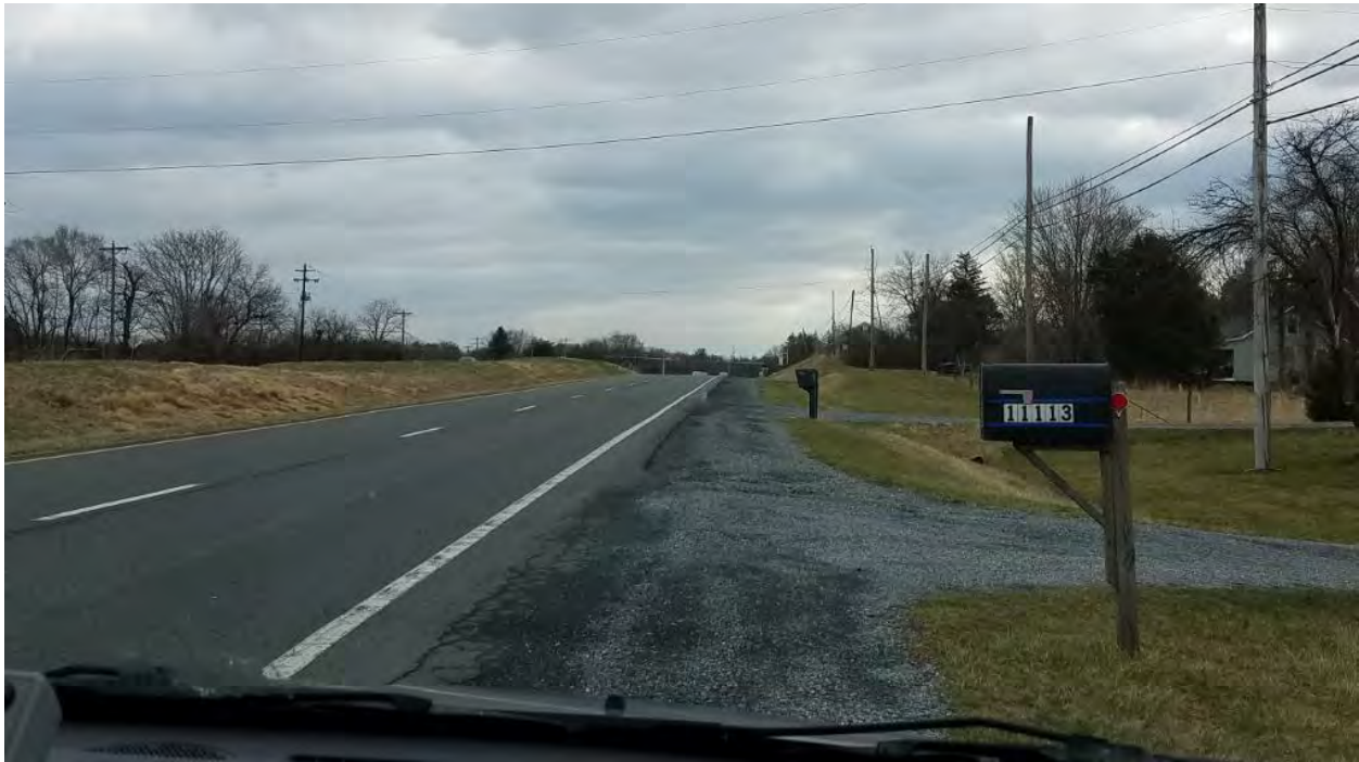
Slight Crest Vertical Curve Eastbound
