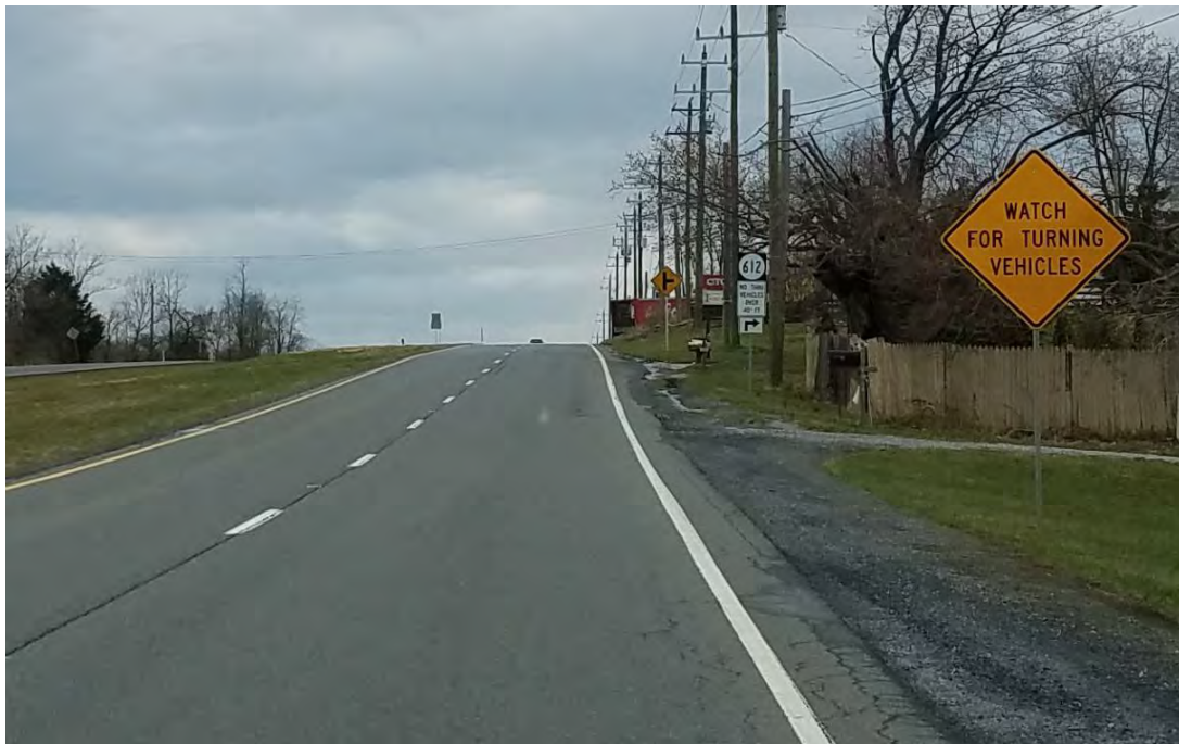
Route 7 westbound approaching Rt 612
