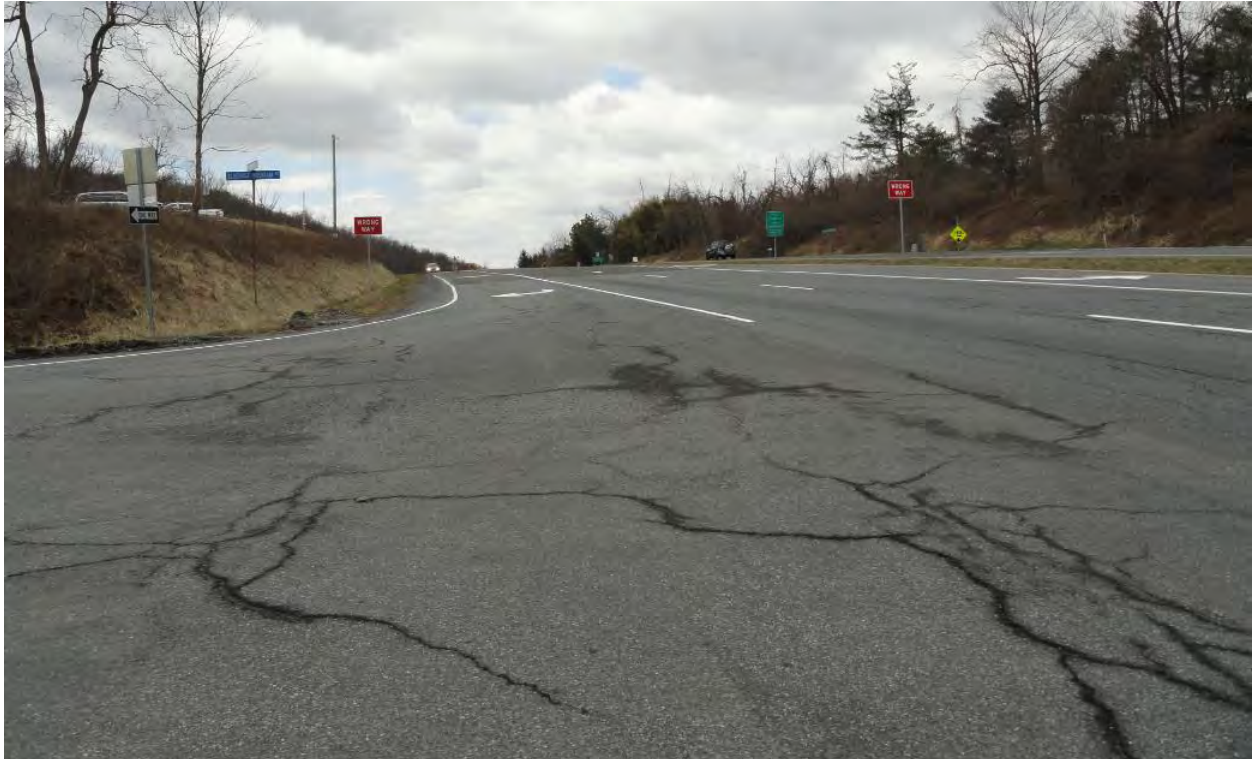
Sight Distance looking east from Rt 601
