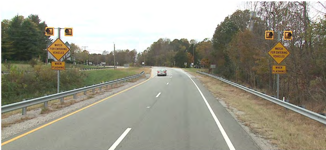
Example of Dynamic Warning Flashers
