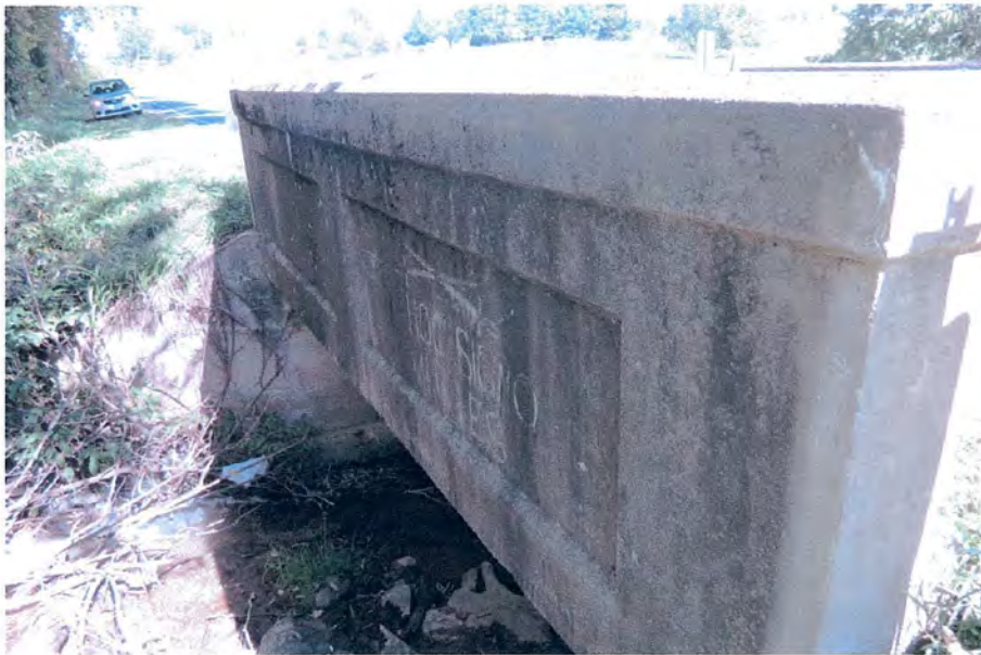
Bridge#6045, looking northeast at "HOC SIGNO VINCES" inscription
