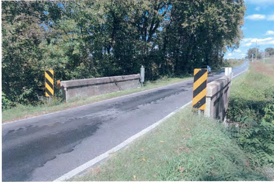
Bridge#6045, looking northwest
