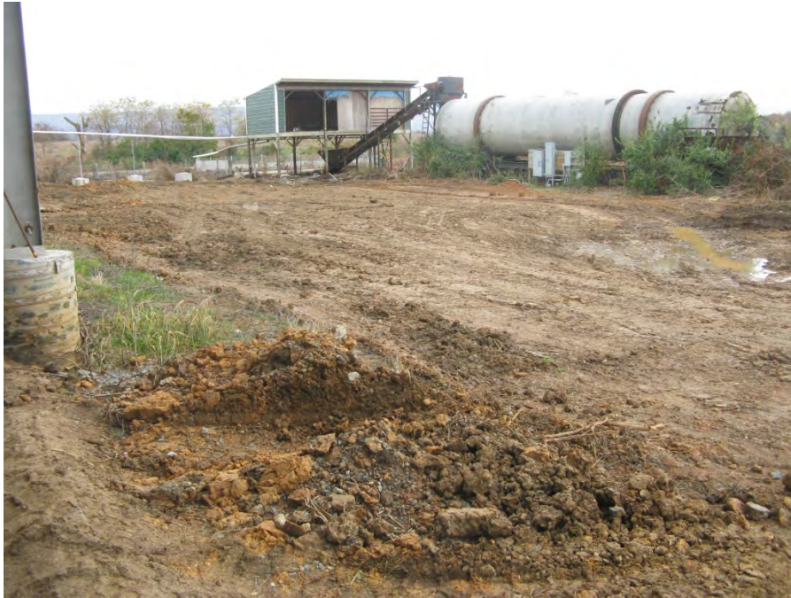
Grading around separator building complete
