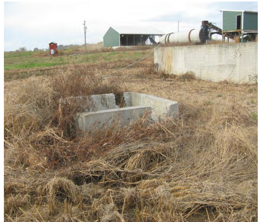
Overflow in catchment basin to manure storage pit
