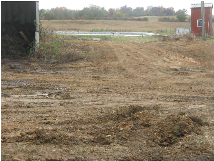
grading around new mortality building complete
