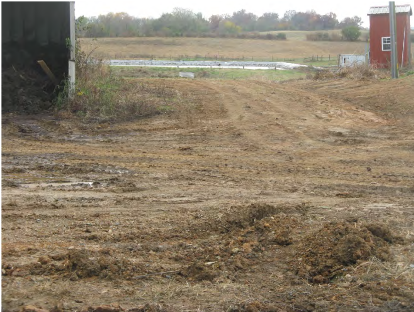
grading around new mortality building complete
