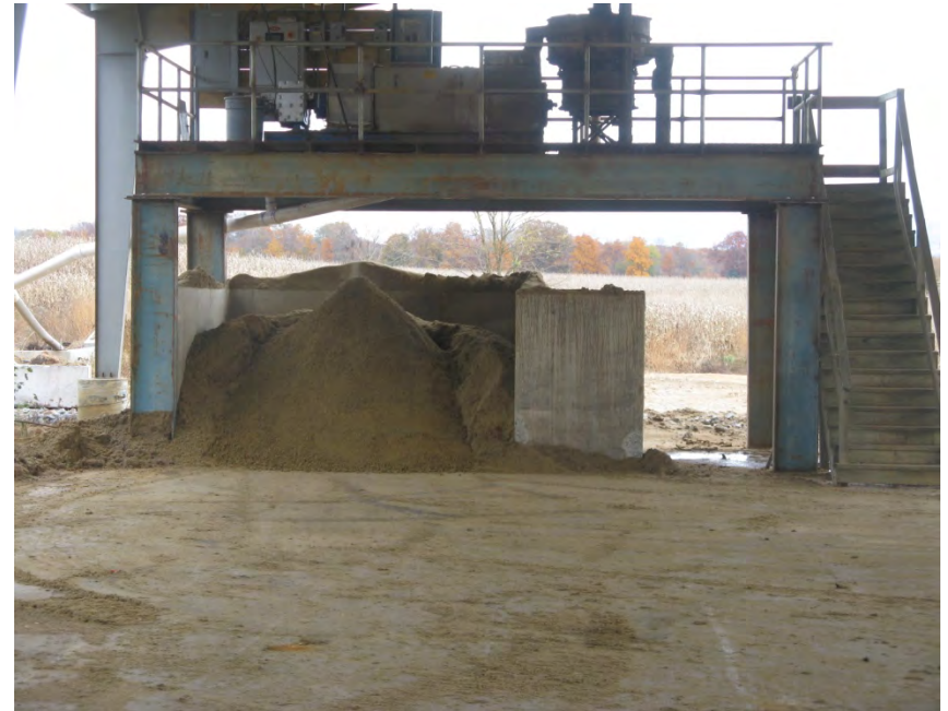
separator relocated and in operation
