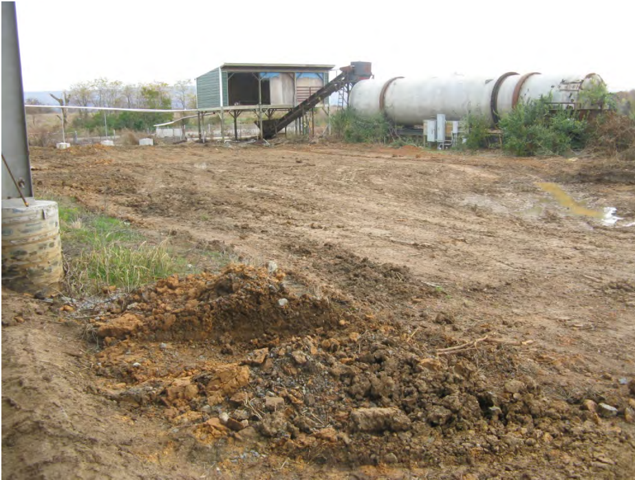
Grading around old separator building complete
