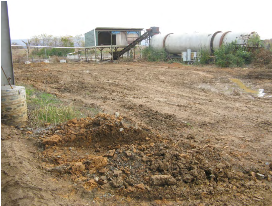
Grading around old separator building complete
