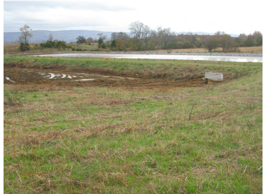
brush cleared from settling basin
