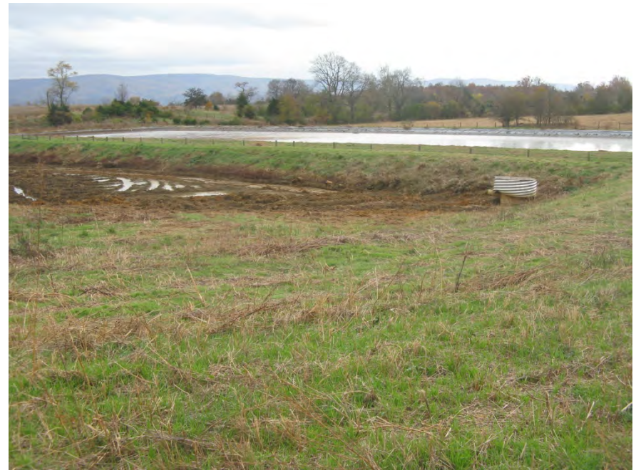
brush cleared from settling basin
