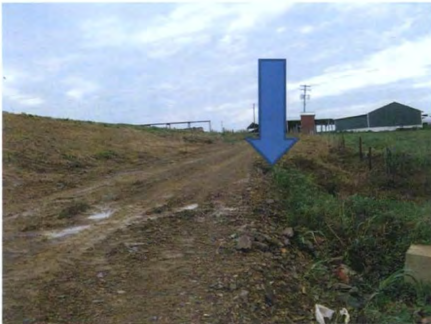
access road to manure storage pits graded – silt fence to be installed (arrow)to direct stormwater away from monitoring well #1
