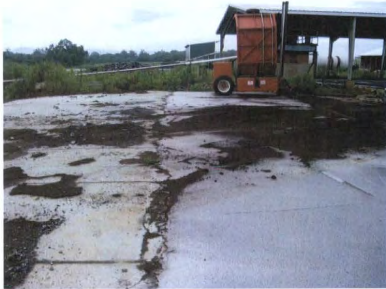
Concrete added to area between compost building and old sand trap
