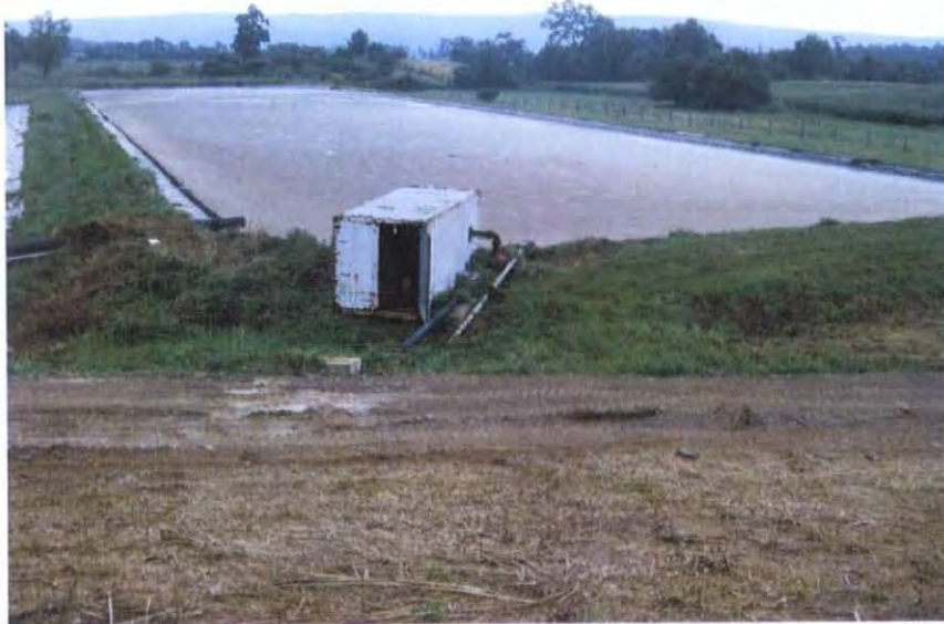
Pump house for pumping flush water To flush tanks from manure pit #1 Also, the manure storage pit is at capacity -18 inch freeboard
