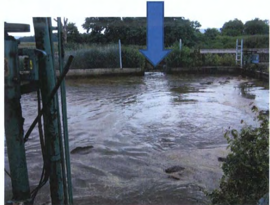
Spill way from reception pit to settling basin
