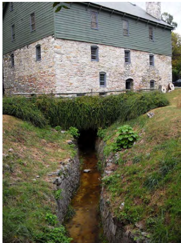
Burwell-Morgan Mill. Source: NSVRC, 2013
