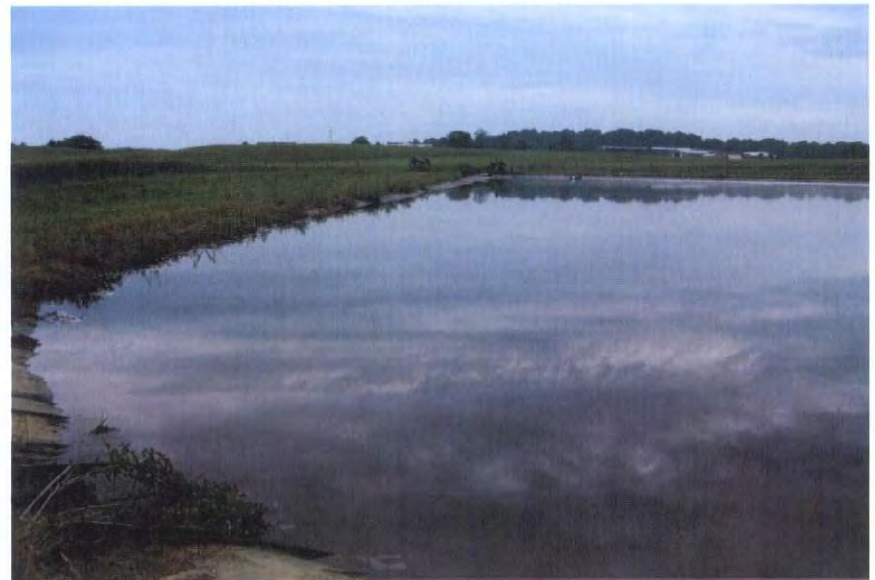
Second manure storage pit - 18 inch free board
