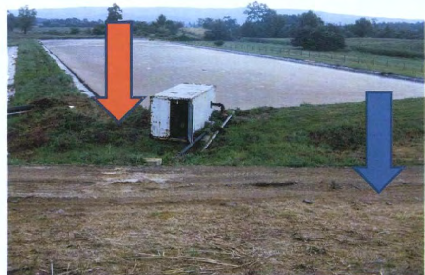
swale to be installed (blue arrow)to direct stormwater from access road away from monitoring well #1 (red arrow)
