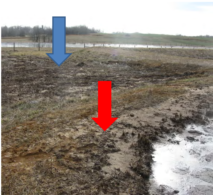
another view of overflow of catch basin berm ( red arrow), and area below the berm where manure has accumulated (blue arrow)
