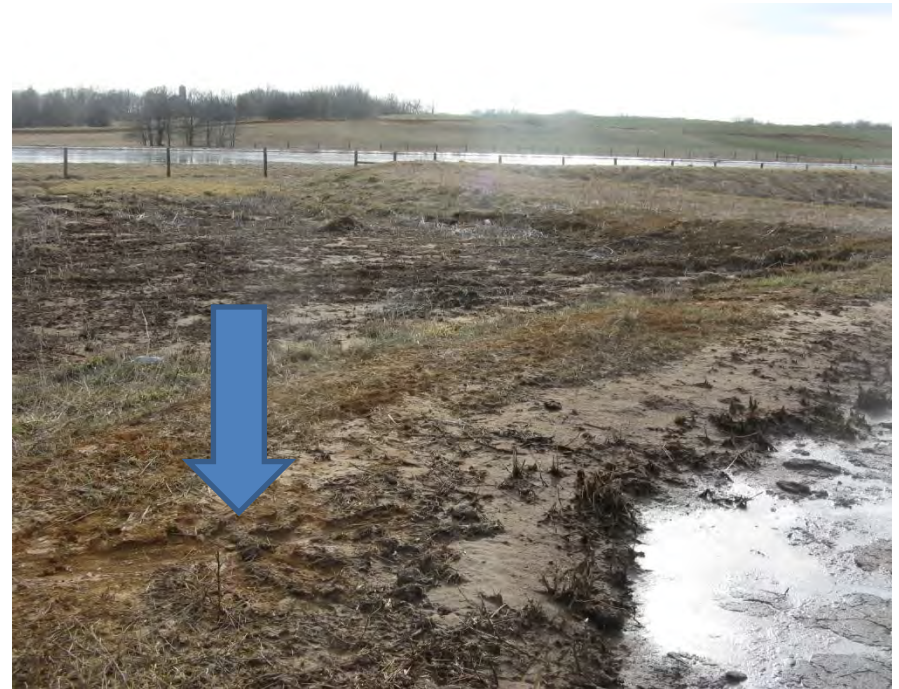
manure overflow from catchment basin arrow show berm that was breached and channel of overflow
