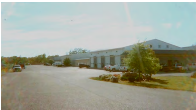
Warehouse Condominium Bays
