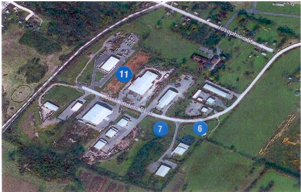
Clarke County Business Park
