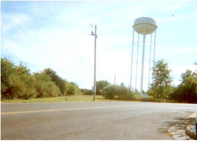
Water Tower Site
