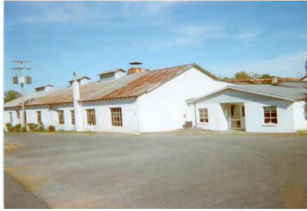
Vacant Industrial Building in 300 Block of First Street
