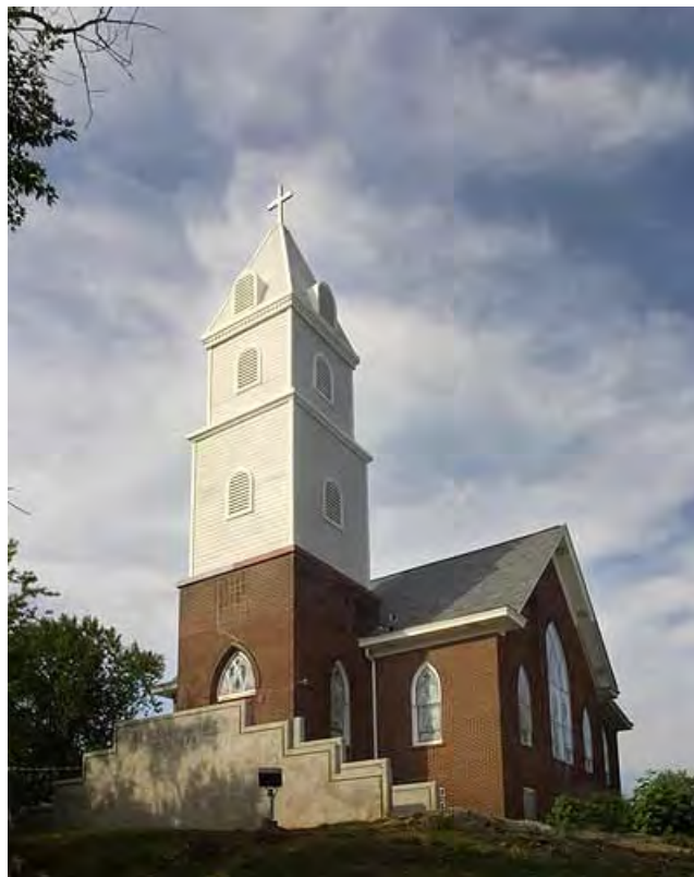
Example of a well-designed bell tower WCF
