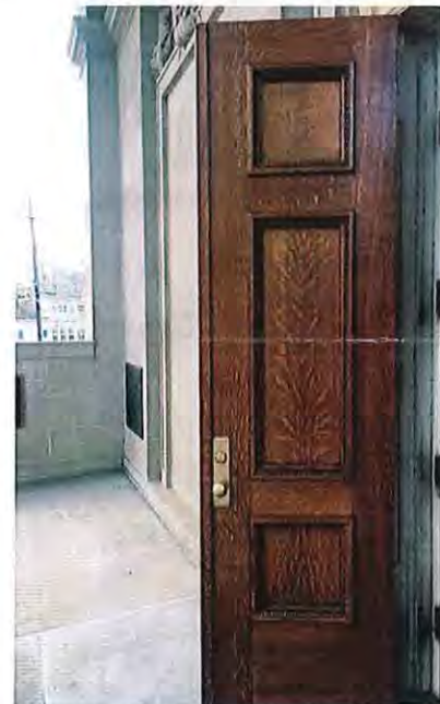
The exterior door at Handley Library was refinished during January.
