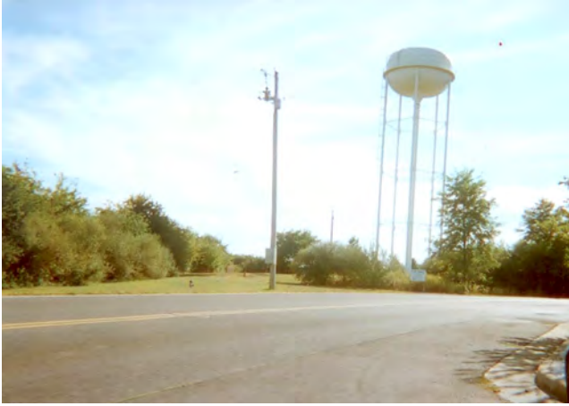
Water Tower Site
