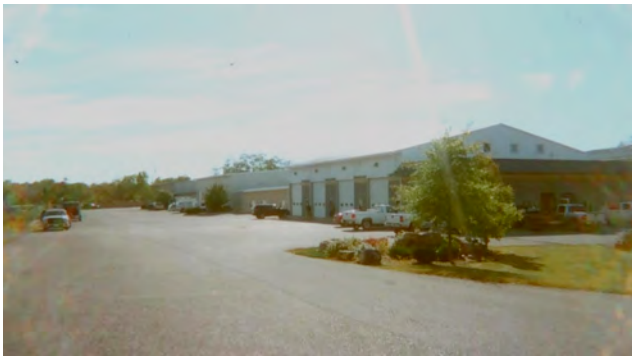
Warehouse Condominium Bays
