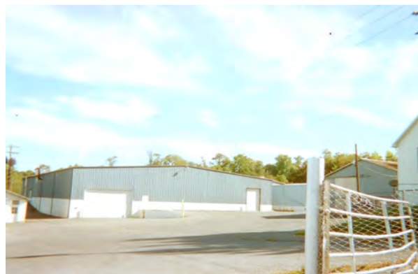
Good Warehouse Space in 300 Block of First Street
