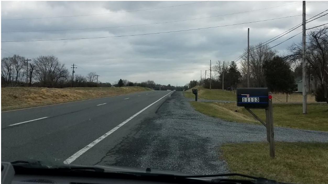
Slight Crest Vertical Curve Eastbound
