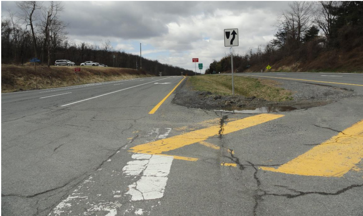
Sight Distance looking east from crossover
