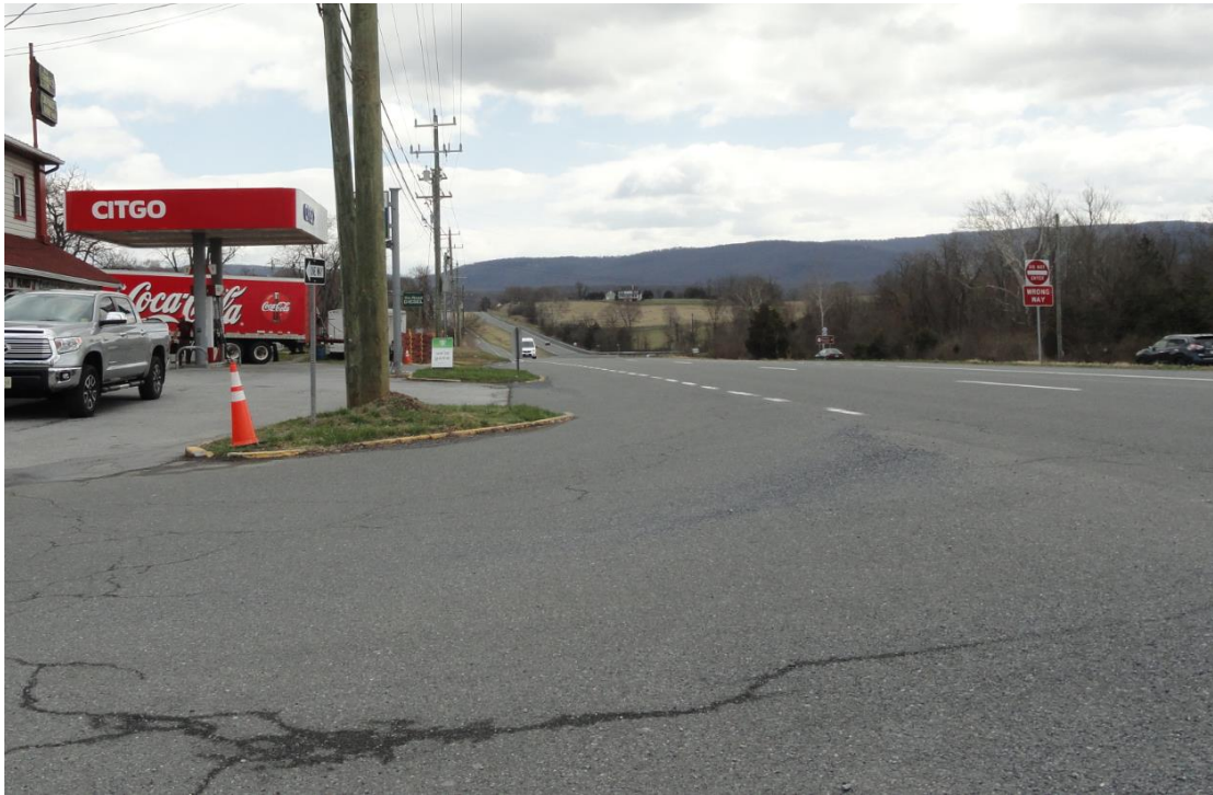
Sight Distance, Rt 612 Looking to the east in the westbound lane
