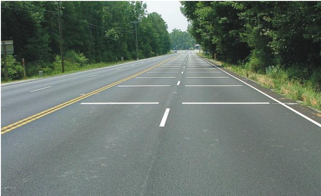
Example of Optical Speed Bar Markings for westbound Route 7
