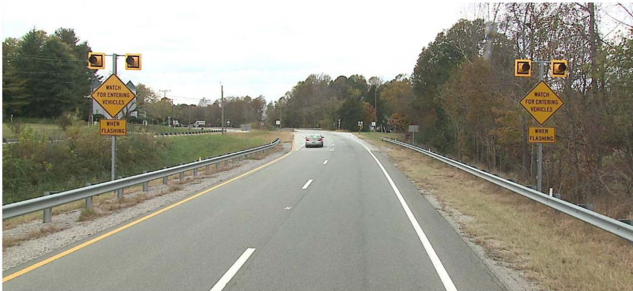
Example of Dynamic Warning Flashers
