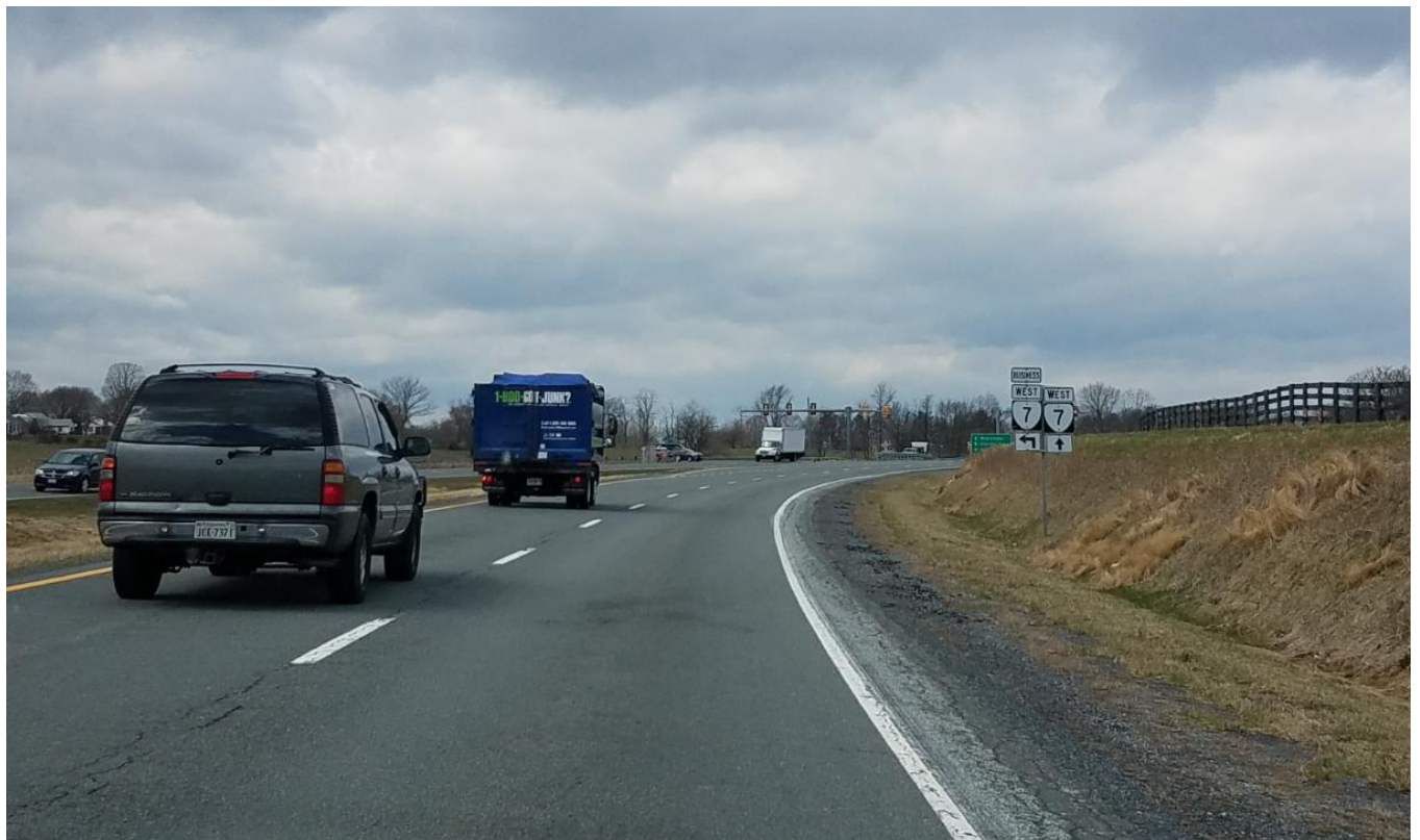
Route 7 westbound, signs blocking signal heads
