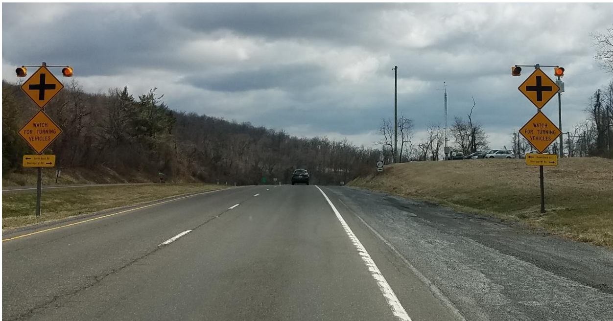
Route 7 eastbound crest vertical curve hiding intersection
