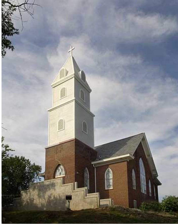
Example of a well-designed bell tower WCF
