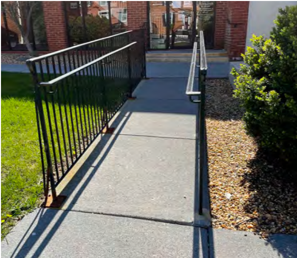
The ramp connecting the N. Church Street sidewalk with the Old Courthouse building has a slope steeper than required by ADA.
