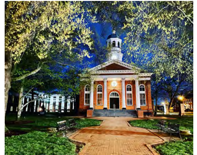
Loudoun County Courthouse, VA
