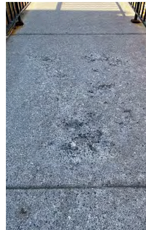
Pavement spalling
