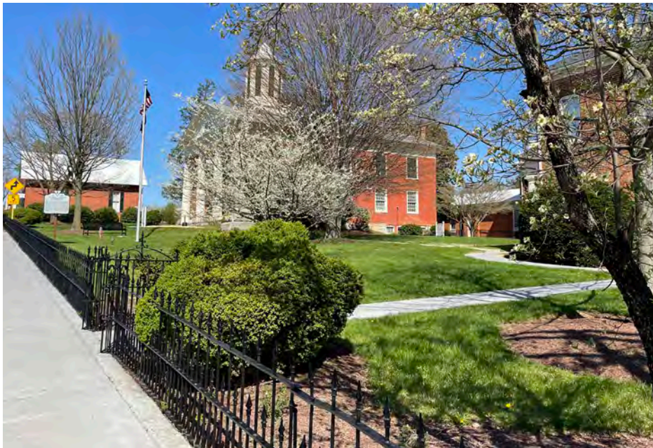
Pedestrian access along N. Church St. through the historic iron picket fence. Both gated entrances are flanked by boxwood shrubs, with concrete walkways leading to the Sheriff's Office and to the Old Courthouse building.
