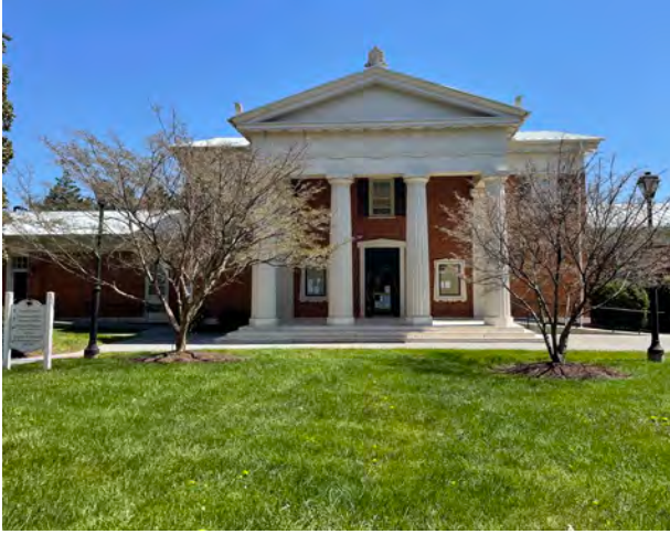
Open lawn areas with trees frame the historic buildings and provide a sense of simplicity, austerity, and security. In the right-hand side of this image, more overgrown shrubs block the view of the building.
