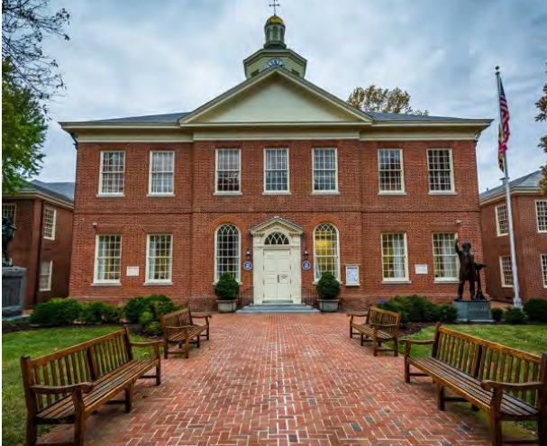
Talbot County Courthouse, MD
