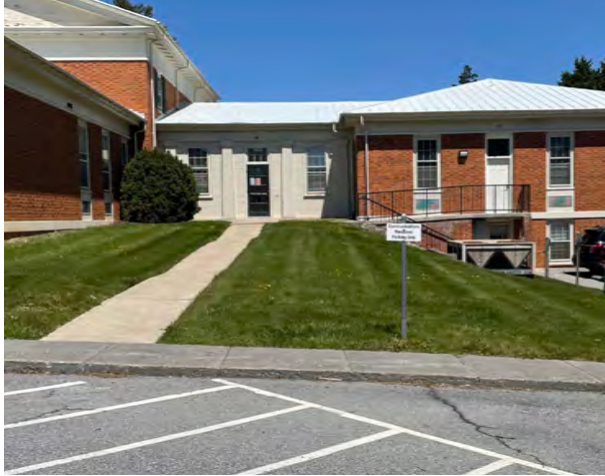
The prisoner escort route from the rear of the New Courthouse building has a sloping sidewalk with one requiring an ADA ramp.
