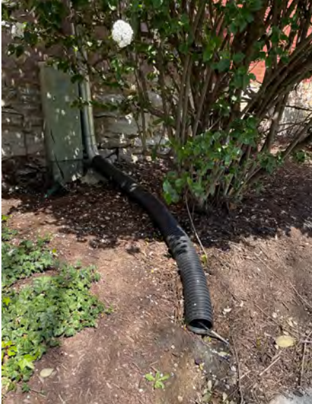
A downspout on the South side of the Old Courthouse building (left) and at the northwest corner of the Sheriff's Office building (right) drain directly into plant beds and cause erosion onto walking surfaces.
