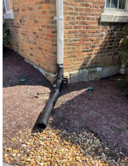
A downspout on the South side of the Old Courthouse building (left) and at the northwest corner of the Sheriff's Office building (right) drain directly into plant beds and cause erosion onto walking surfaces.
