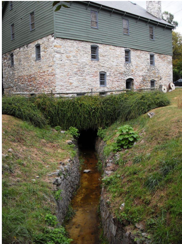
Burwell-Morgan Mill. Source: NSVRC, 2013
