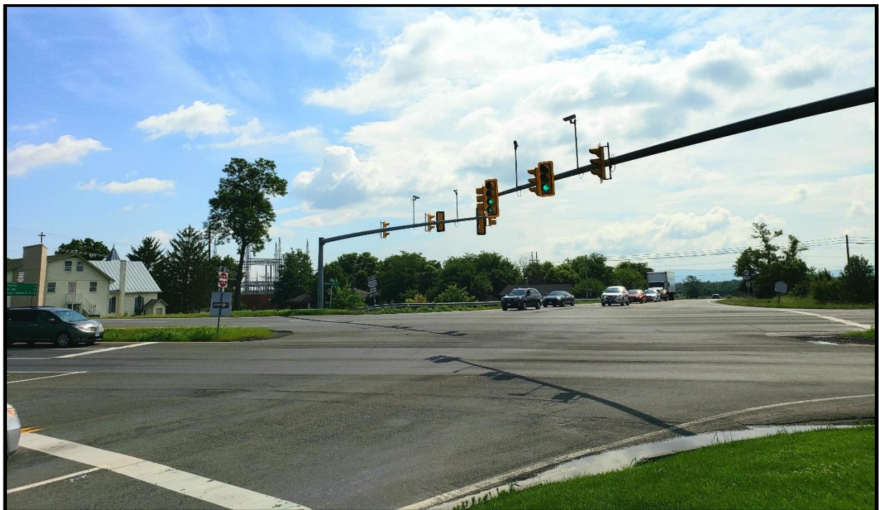
Figure 2 – View of intersection towards northeastern quadrant
