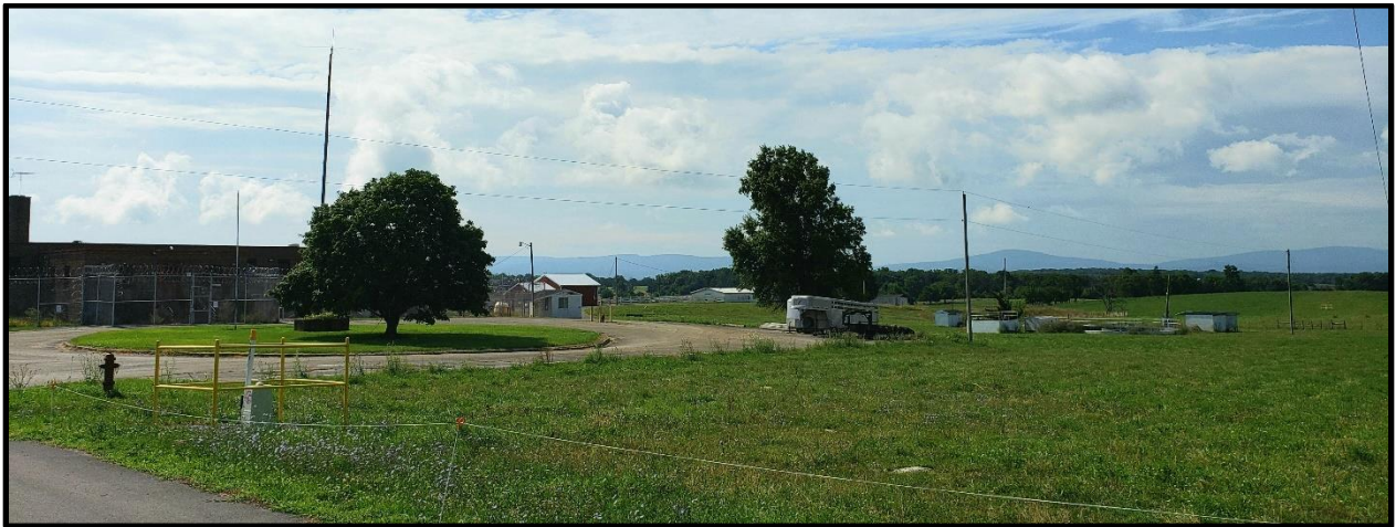
Figure 8 – Vacant former Department of Corrections facility and sewage treatment package plant
