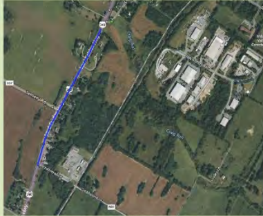
Corridor Study – Lord Fairfax Highway (US 340) between Smallwood Lane (Route 680) and Town of Berryville limits; VDOT 91 st (15 total crashes, 4 injury/fatality)
