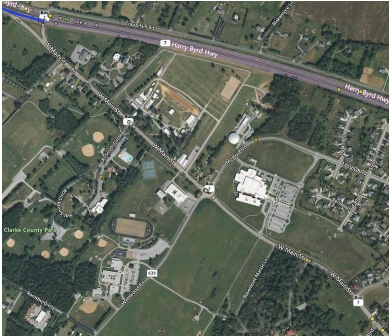
West Main street corridor from Harry Byrd Highway to Hermitage Boulevard
