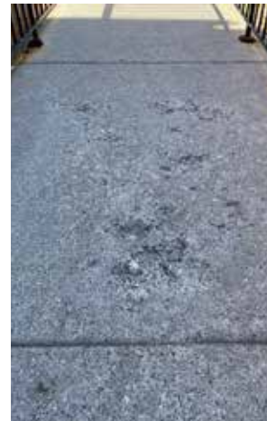
Pavement spalling
