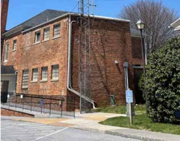
ADA accessible parking spaces are provided at an entrance between the Sheriff's Office and the New Courthouse building.
