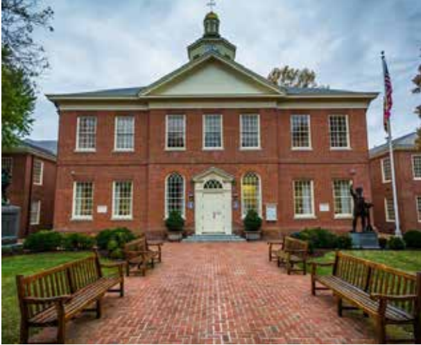
Talbot County Courthouse, MD
