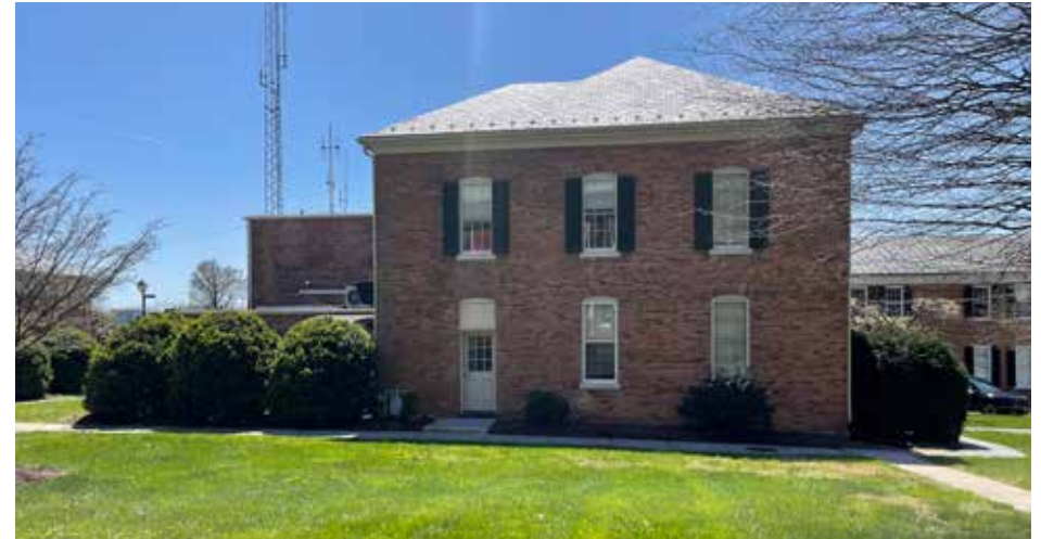
The character of the Courthouse Green is marked by lawns, mature trees and large shrubs at the building foundations. Sheriff's Office shown in background.
