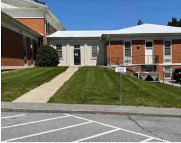
The prisoner escort route from the rear of the New Courthouse building has a sloping sidewalk with one requiring an ADA ramp.
