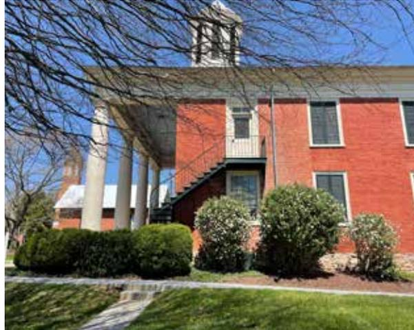
Against the Old Courthouse building, a variety of large shrubs block the view of the building, trap moisture behind the walls, and impede foot traffic along the narrow sidewalk.
