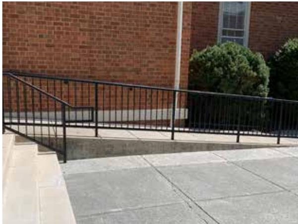
The ramp connecting the ADA parking spaces at the southeast to the New Courthouse building has a sloping sidewalk with one section steeper than required by ADA.
