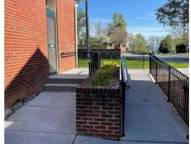
The ramp connecting the northwest vehicle drop-off with the Old Courthouse building has a slope steeper than required by ADA.
